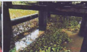
Picture showing impacted area.
